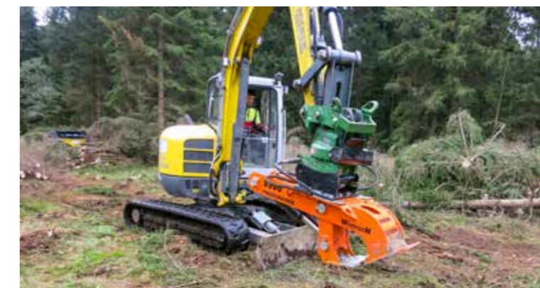
Usage in loose, sandy and erosion-prone soils.
