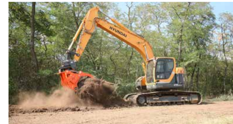
Clearing and caring of large areas.
